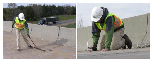
Figure 2.6. Chain Dragging (Left), and Hammer Sounding (Right) [22]
