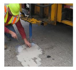
Figure 3.6. Extraction of Cores
