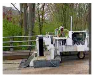
Figure 2.12. Hydrodemolition Machine [45]
